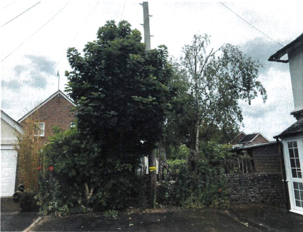
Pictures represent only part of the damage
