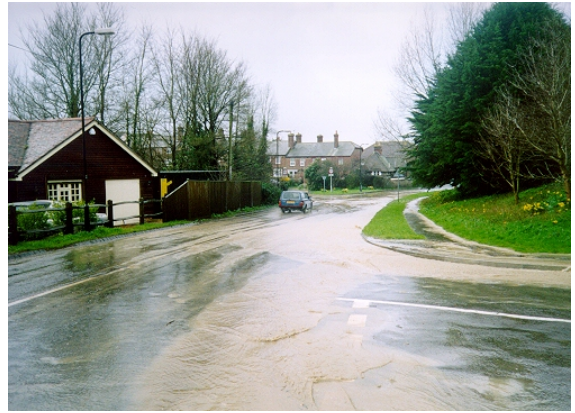
Dappers Lane surface water flooding photographs 2002. Runoff from adjoining land and frequently flowing down both sides of the road.
