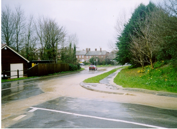
Dappers Lane surface water flooding photographs 2002. Runoff from adjoining land and frequently flowing down both sides of the road.
